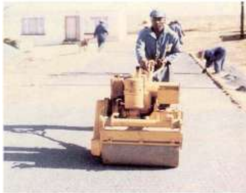
Figure2.9 Compaction of the aggregate
