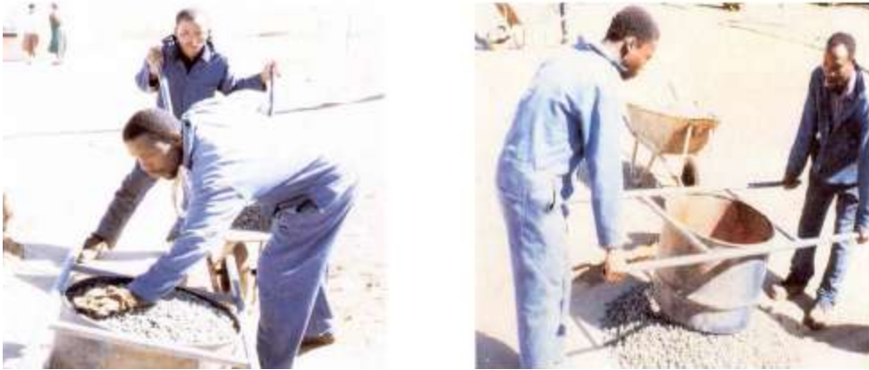
Figure 2.8 spotting of aggregate
