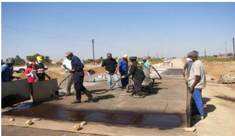
Figure 2.3 spraying of tack coat with a motorized hand sprayer
